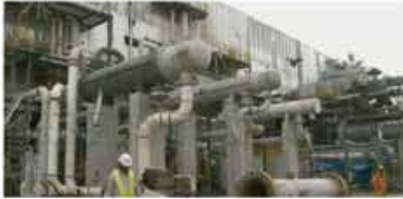
Dangote Petrochemicals Project, Dangote FZ, Ibeju-Lekki, Lagos.
